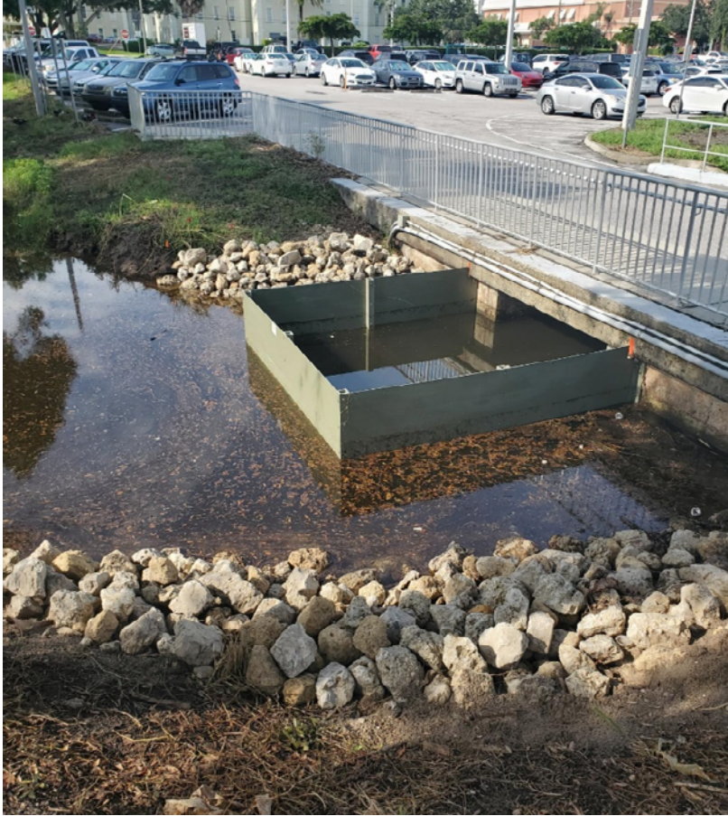
South Channel – Skimmer Structure to Hudson Bayou
