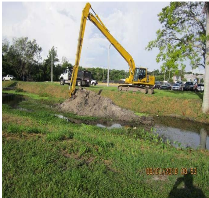
North Channel – Sediment Sump Excavation
