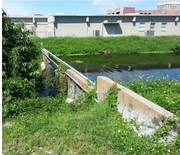
Sarasota High School North Channel Weir
