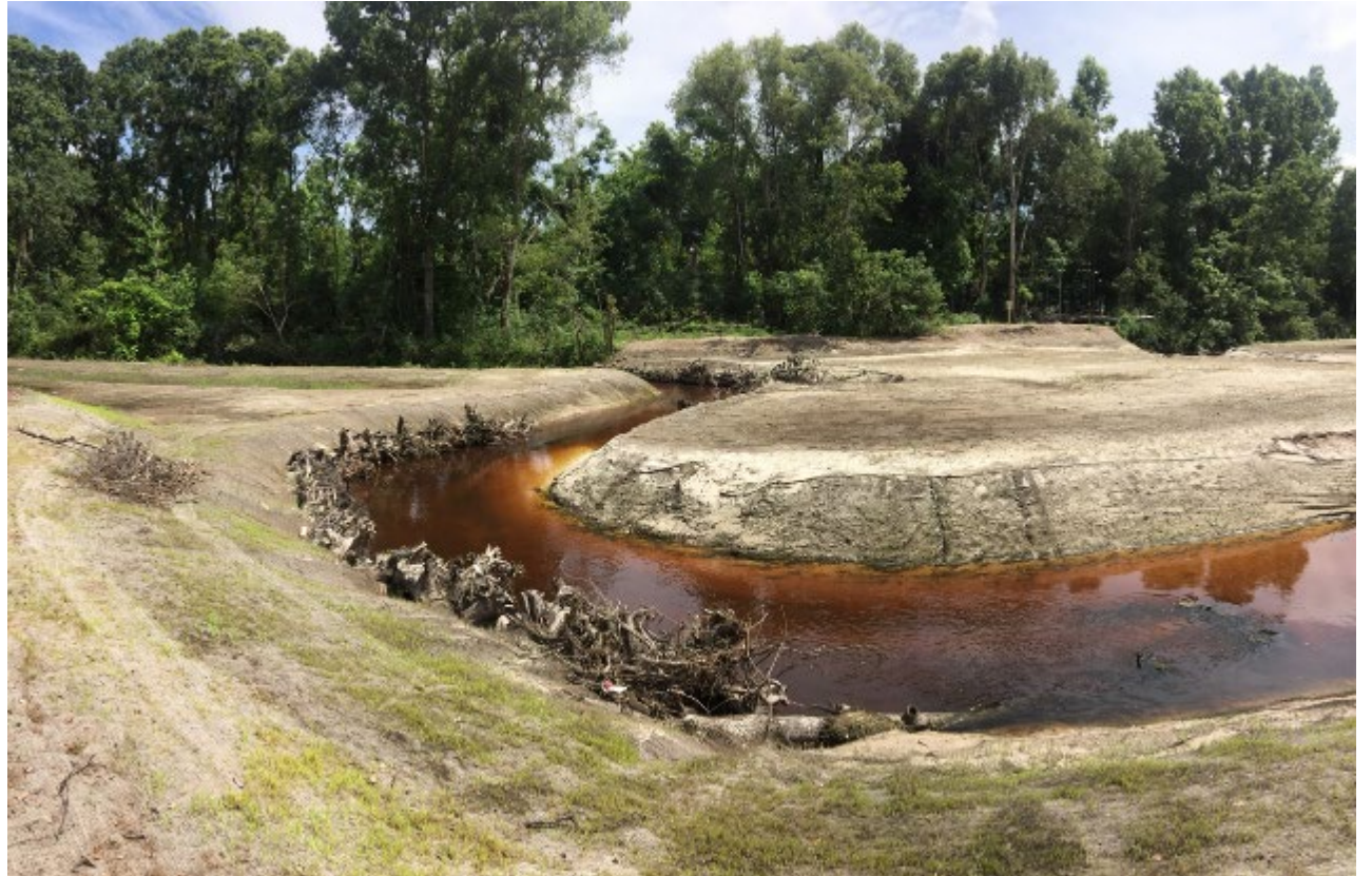
Edwards Bottomland Project – ongoing construction undamaged by flood
