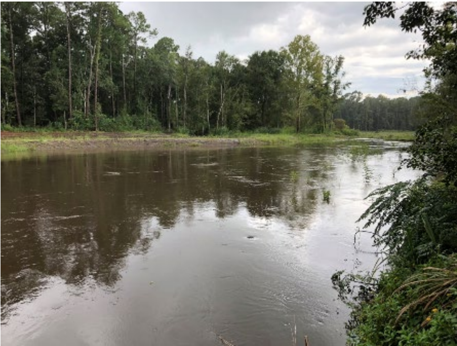
Edwards Bottomland Project – flood under construction
