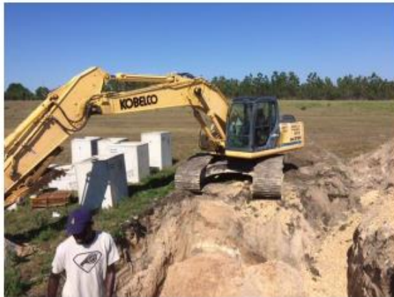
Excavation of BMPs
