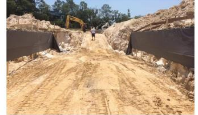
Placement of impermeable liner
