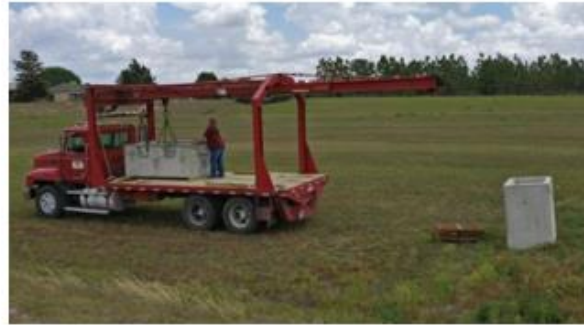
Delivery and placement of vertical reactors
