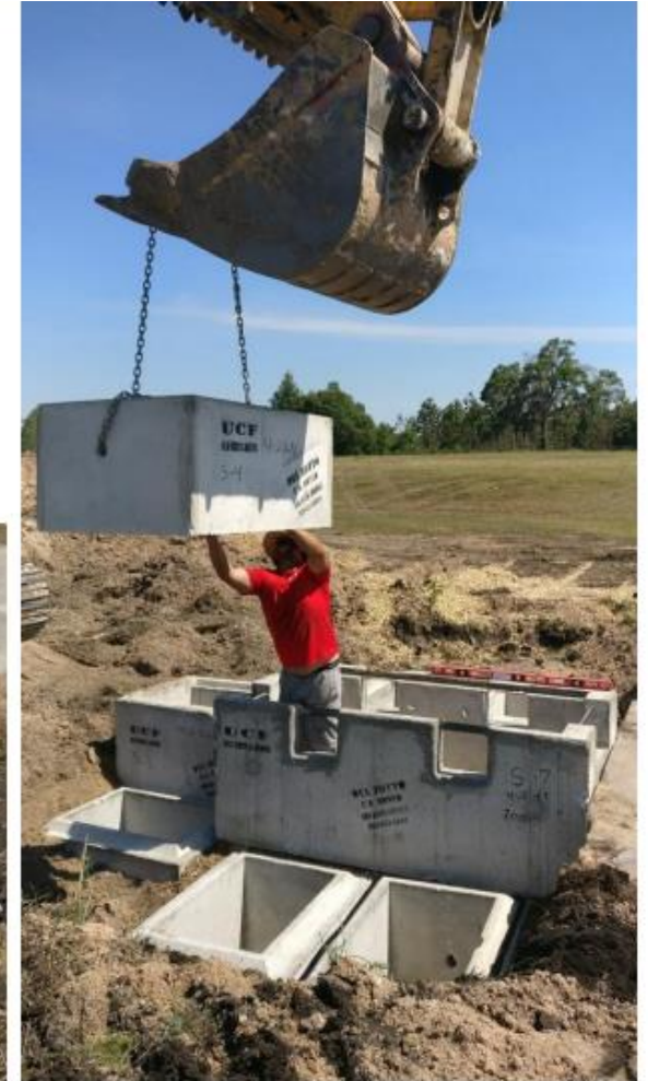
Delivery and placement of vertical reactors
