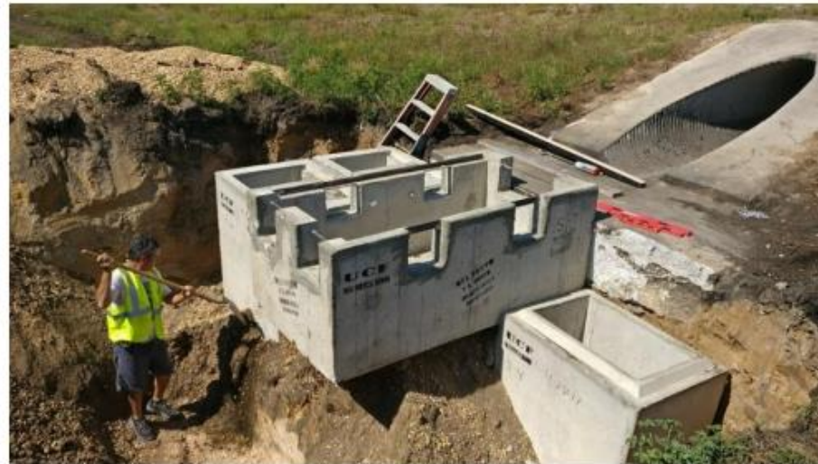
Delivery and placement of vertical reactors
