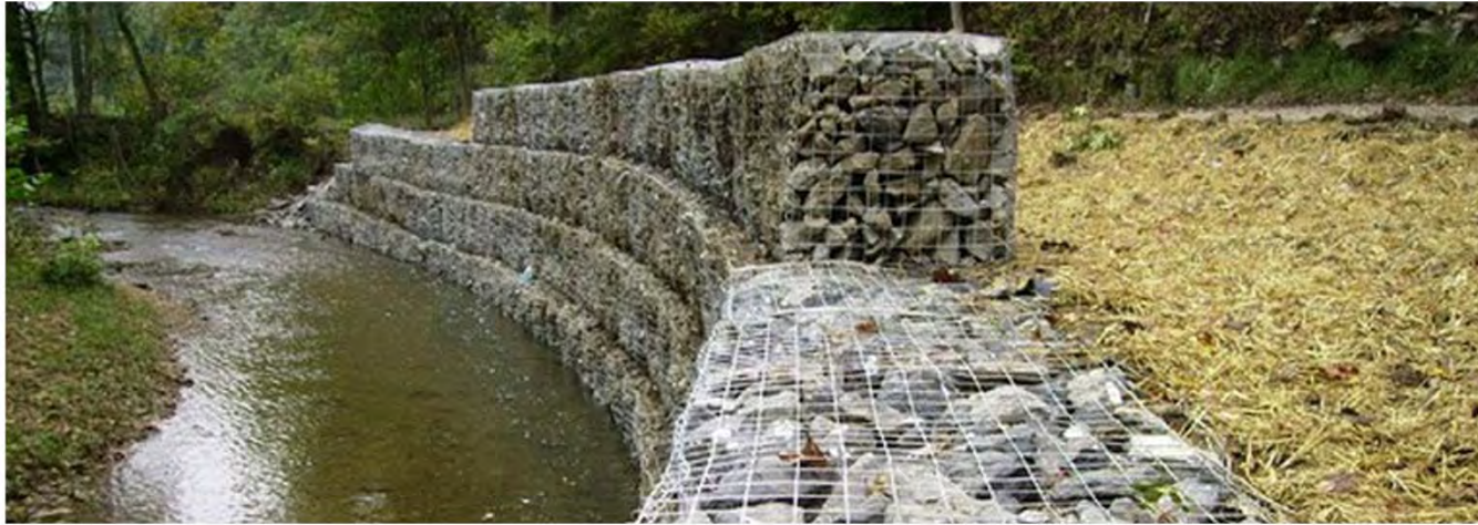
i. Photo credit: http://gabion1.co.uk/river-bank-protection/
