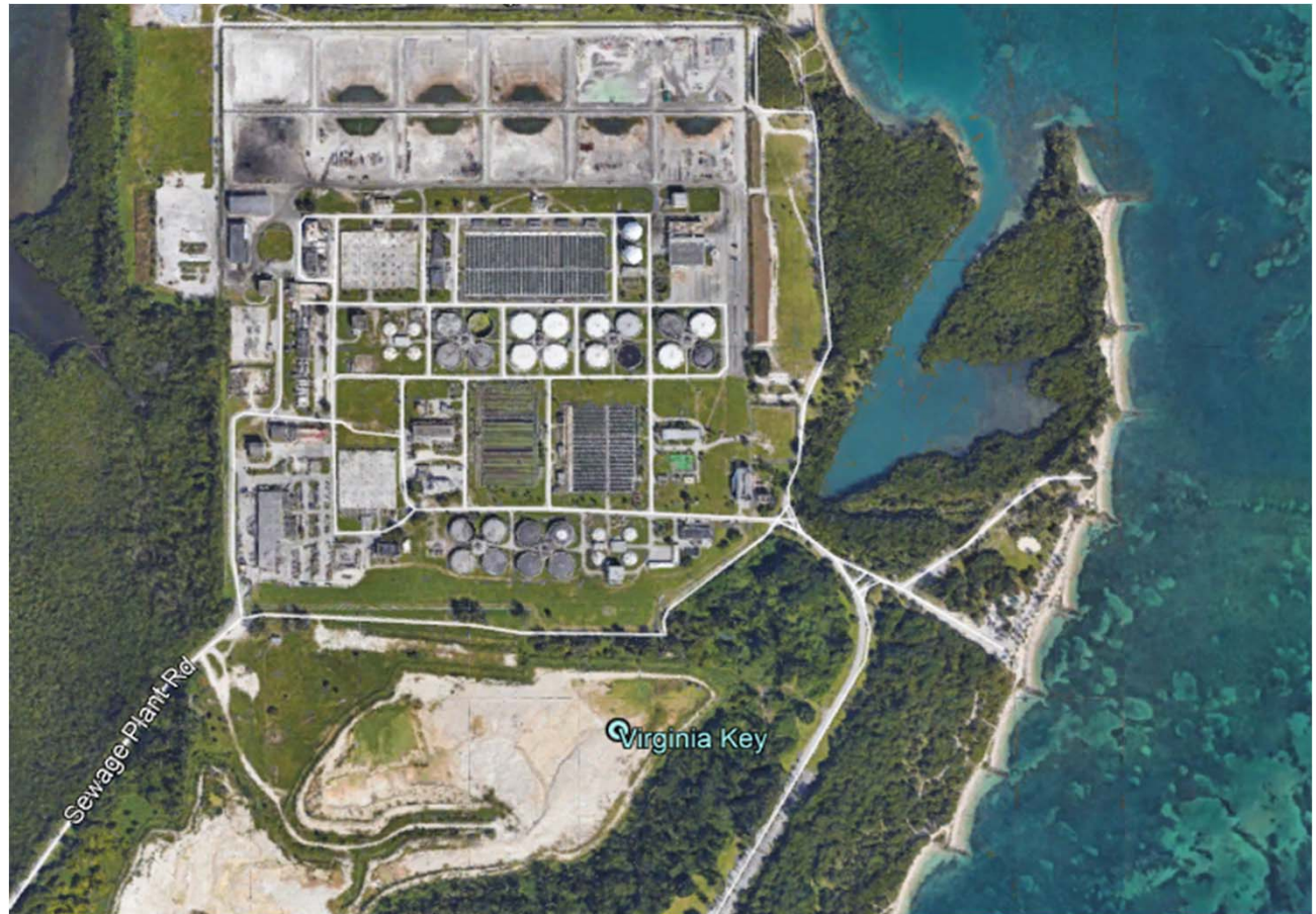
Wastewater Plant on Virginia Key, Miami
