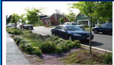
Bioswales are essentially rain gardens placed in long narrow spaces such as the space between the sidewalk and the curb.
